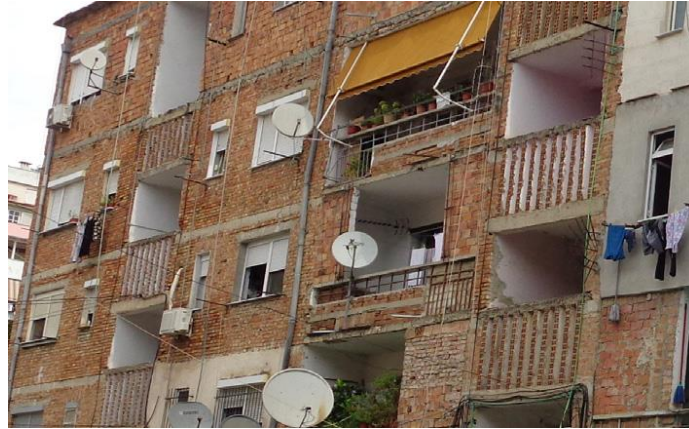
Figure 4: Picture of the existing façade
