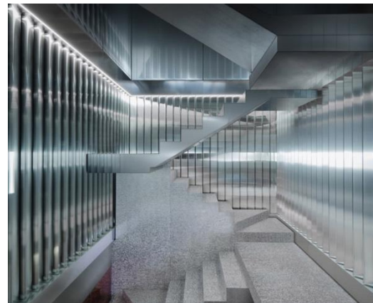
Figure 3: Left: OMA, Milan, Italy, interior and exterior cladding. Right: OMA, Paris, France, interior cladding, the steps on the lower section are made from aluminum foam
