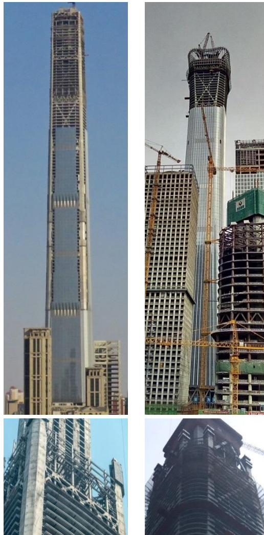
Figure 4. Goldin Finance 117 and Citic Tower under construction
