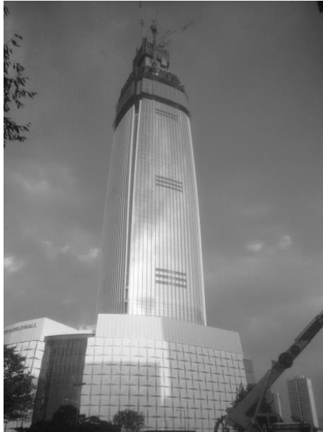
Fig. 2. Lotte World Tower during construction.
