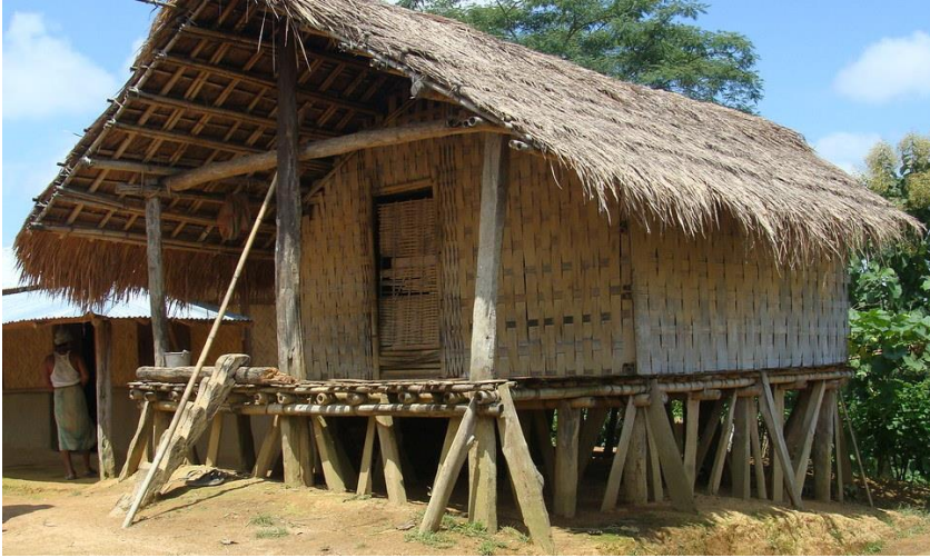
Figure 1: The Traditional Riang living-house. The construction of these types of house generally takes place in the dry season especially in winter since the construction materials like thatch/ timber/ bamboo are collected during winters only.
